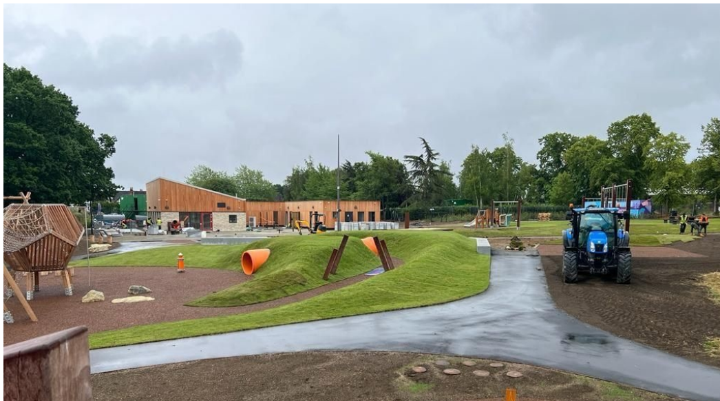
Works are almost complete on the new building and playground.
